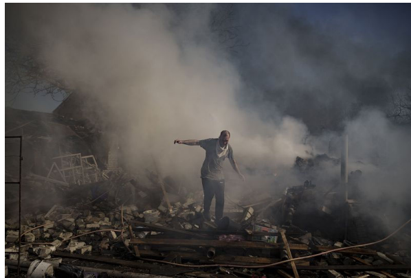
Fig. 3. Destruction in Kharkiv, March 24, 2022 (Felipe Dana/AP) - A man walks through the rubble of a burning building after Russian shelling, recording traces of violence and destruction.
